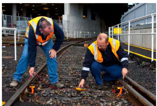
An outer flagman places detonators on a track
